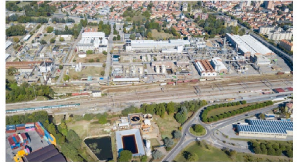
Trinseo Manufacturing Operations, Rho, Italy. Site of future demonstration PMMA depolymerization facility.
